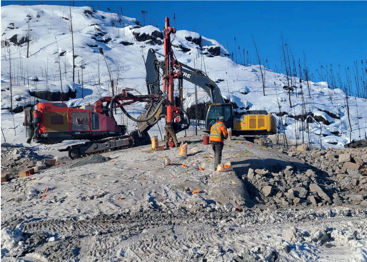
Preparing the blast for the mill foundation
