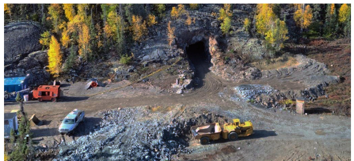
Aerial view - A-Zone mine portal
